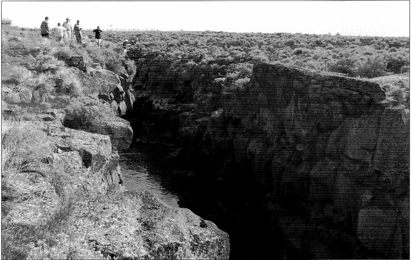
The Kelton Road bridge abutments at the Malad River gorge.
